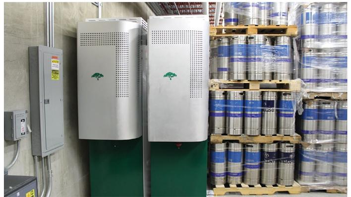
A 30 kW/60 kWh GridSynergy system, located in the basement of Mike Hess Brewing’s North Park brewery, mitigates spikes in power demand caused by daily operations.
