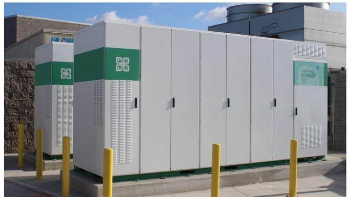
Monitored around the clock from ENGIE Storage's network operations center, Poway's GridSynergy storage systems automatically discharge power to prevent demand spikes at the meter.
